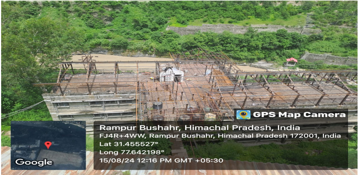
43. Ongoing work for roofing of tribal hostel (Boys).
